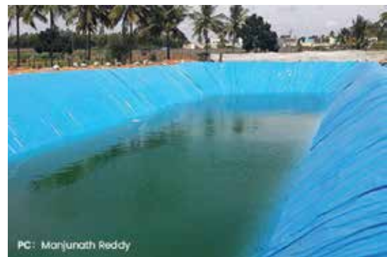
Figure 15. Rainwater harvesting pond
