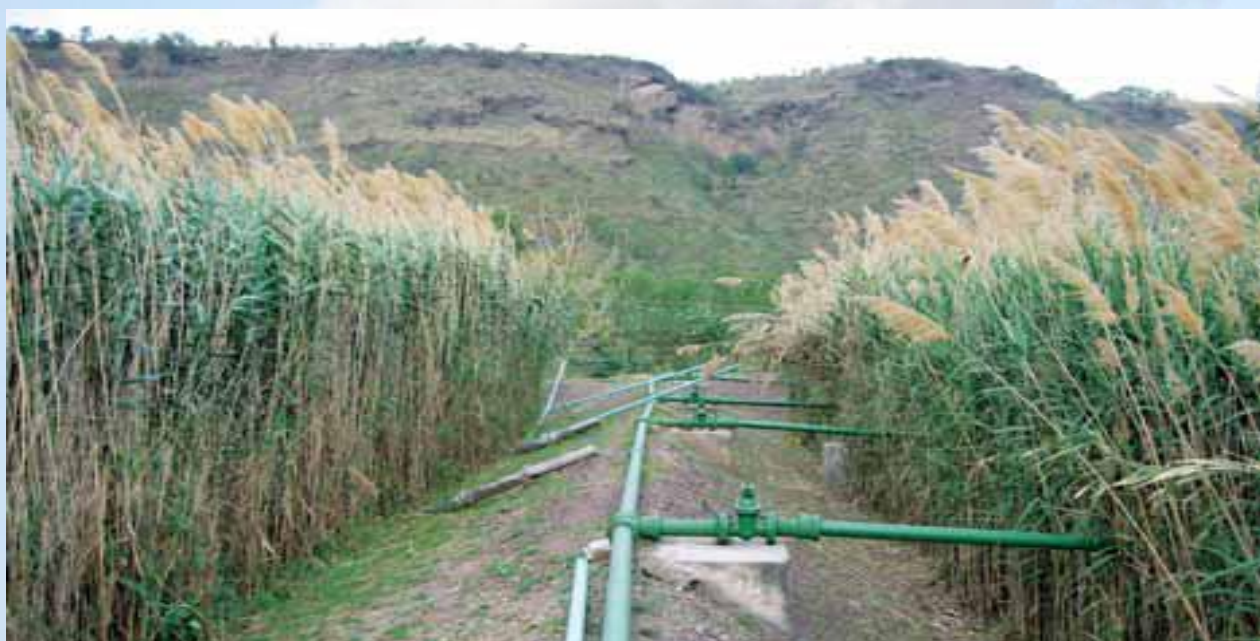
Root Zone Biotech plant at ACC Gagal for waste water treatment
