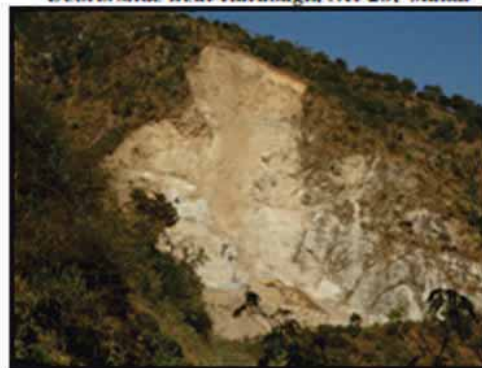
Debris slide near Mandi town ( Due to quarrying)
