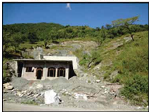
Debris slide near Chirang, NH-20, Mandi
