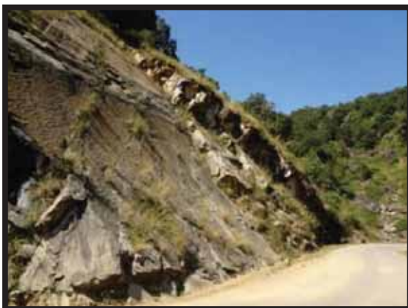
Planar failure observed near Joginder Nagar, Mandi district
