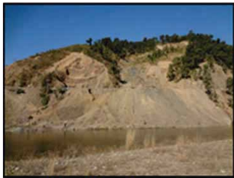
Debris slide near Dadahu, Sirmur
