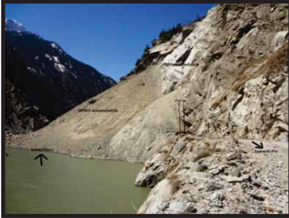
Debris cone over road and river
