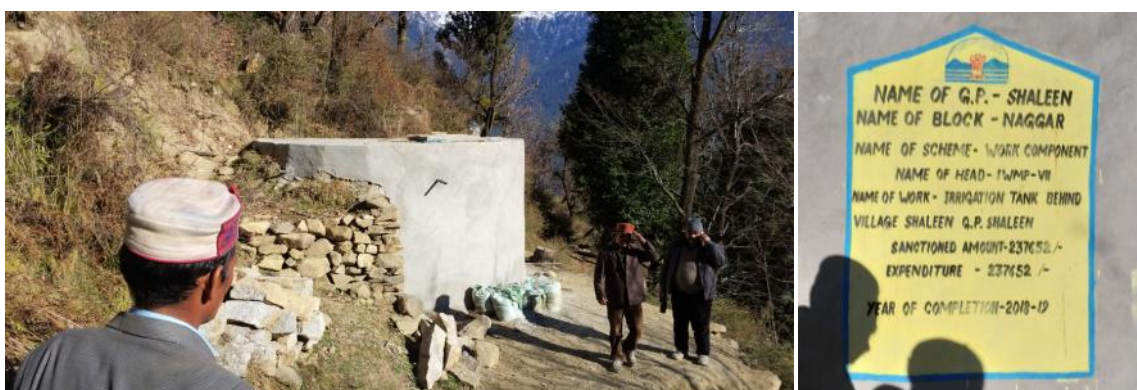
(Storage tank constructed by IPH)
