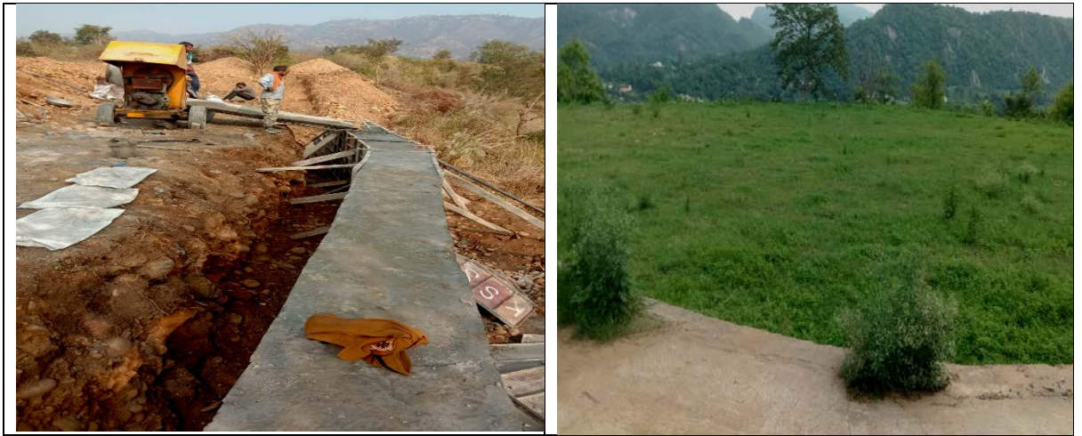
Figure 7 Construction of Eco-Village park at Village Changar Handola, Block Bangana, Una.
