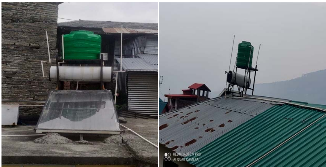
Figure 10 Installation of solar geyser in village Bhanjradu, district Chamba
