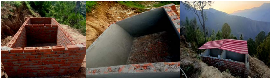
Figure 5 Construction of Farm pond by using traditional method in village Baghalli ,District Shimla, Himachal Pradesh
