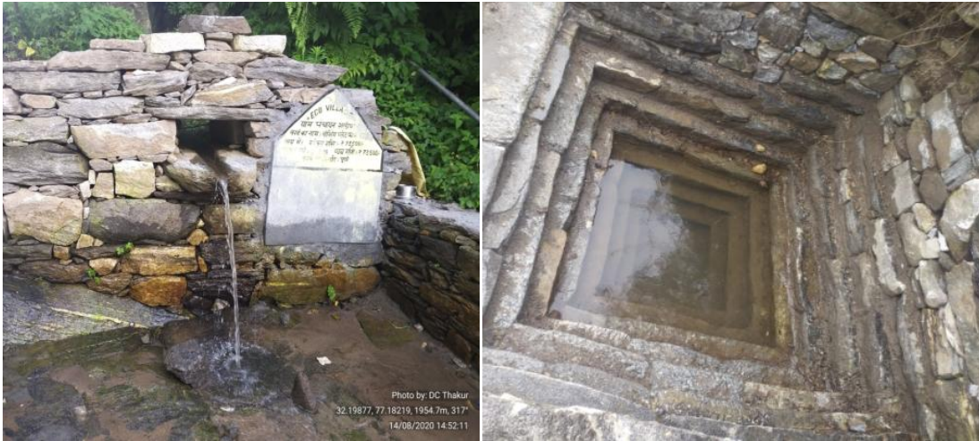
Construction of Bawaries by using traditional method in village Shaleen, Kullu
