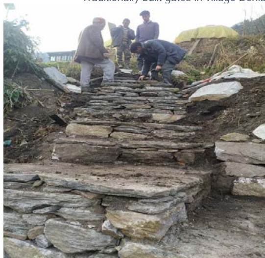
Construction of roads by using traditional method in village Shaleen, Kullu
