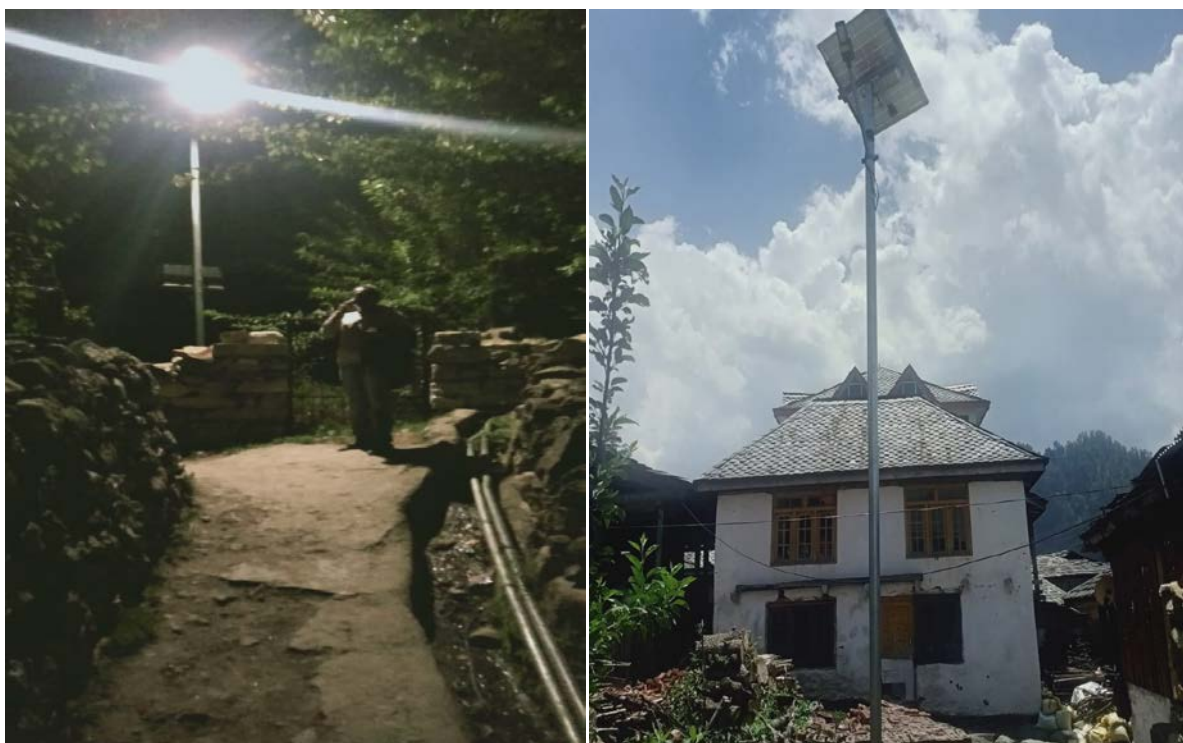
Solar lights installed in village Mahog-Solan , Kamru-Kinnaur and village Baihala, Janjehli, Mandi
