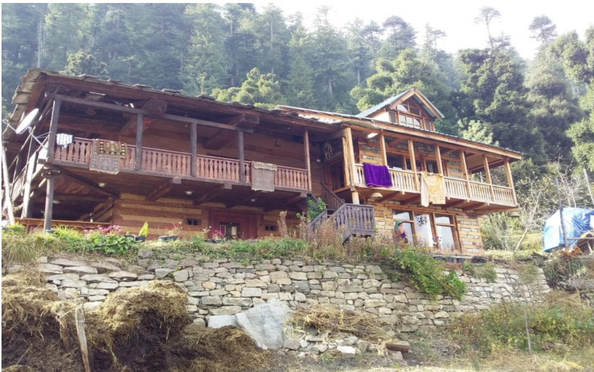
Promotion of building construction by using traditional method Kath-Kuni style in village Shaleen, Kullu
