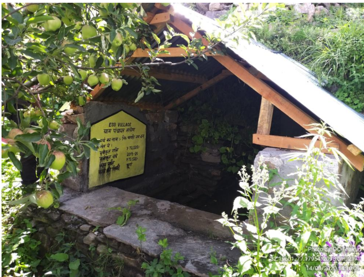
Construction, maintenance and protection of water source in village Shaleen, Kullu
