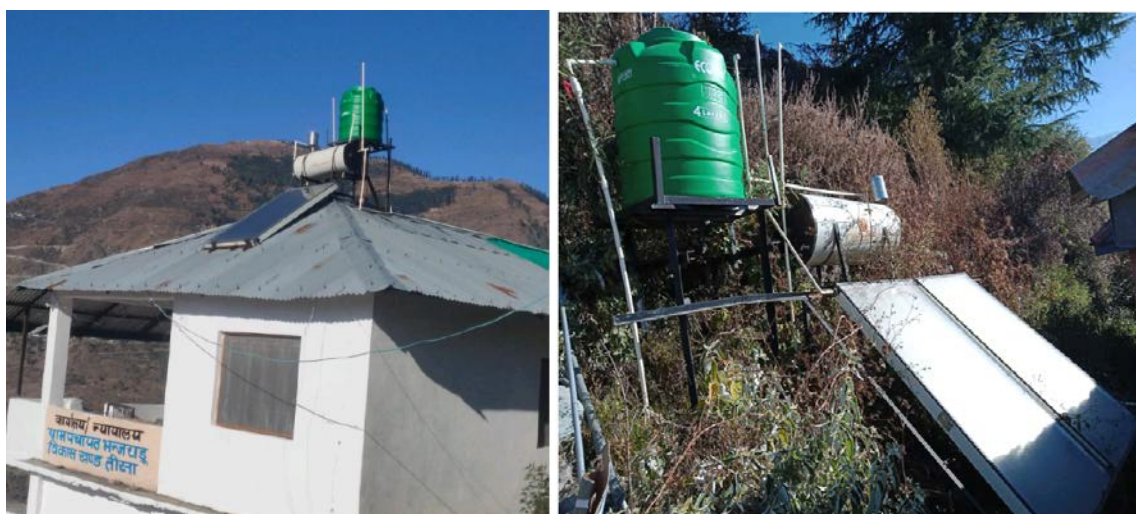
Installation of solar geyser in village Bhanjradu district Chamba
