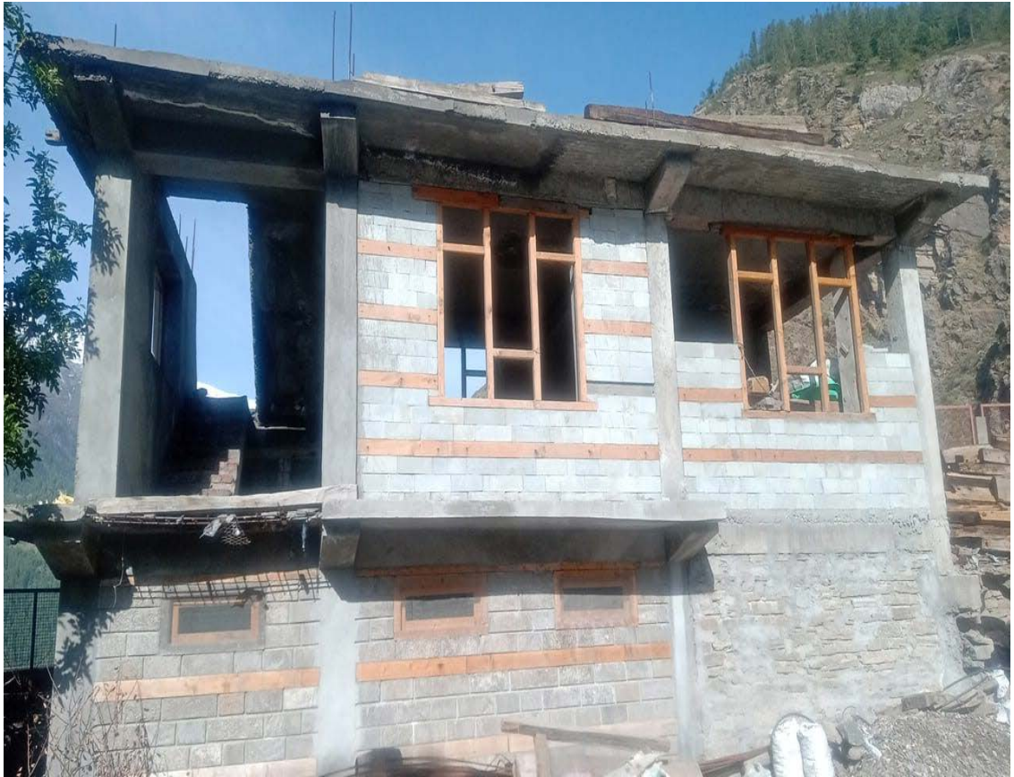
Construction of tourism assistance center in Kamru-Kinnaur
