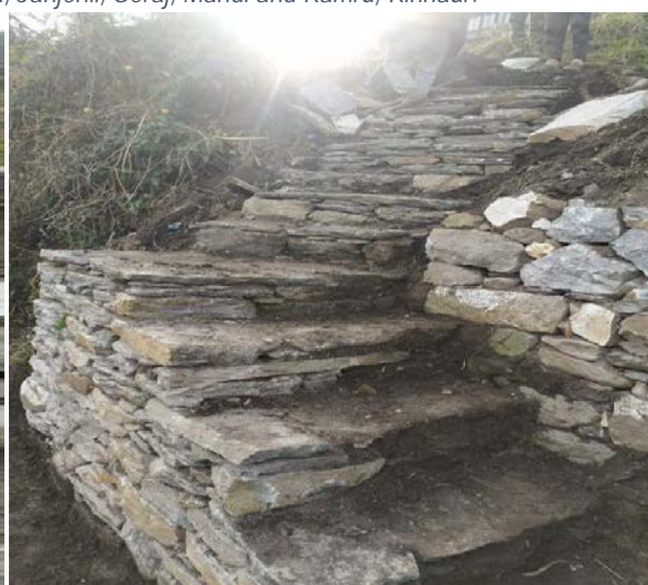
Construction of roads by using traditional method in village Shaleen, Kullu
